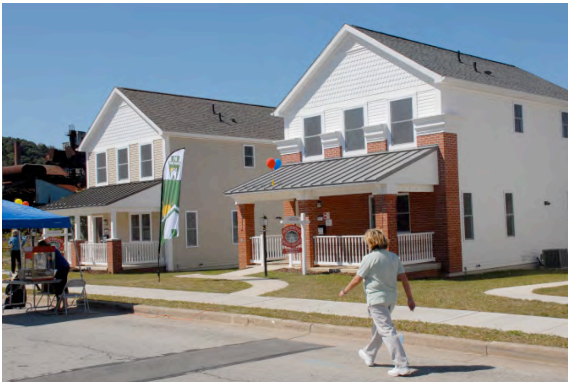
Figure 3. South Sixth Street Project, (Jeanette, PA - Nine New Energy Star Qualified Homes Assisted by PA Home Energy Program, September 2009).
